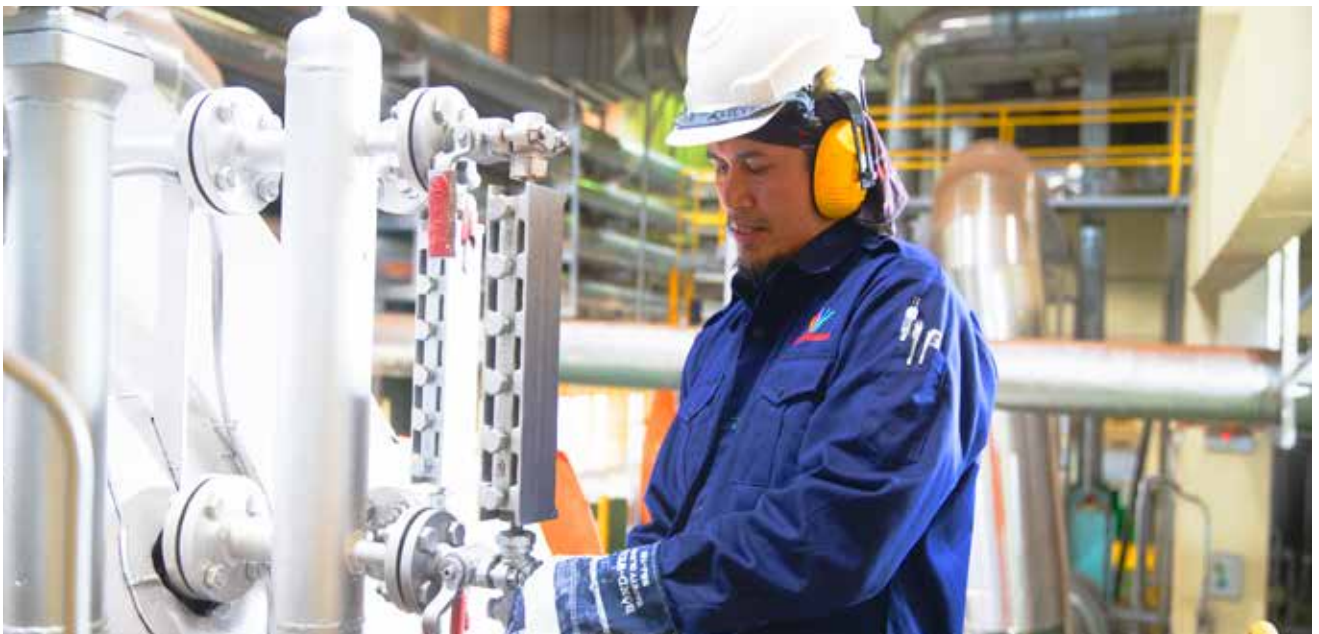
At Genting Malaysia, we place importance on conducting daily inspections of our boiler system to ensure reliability and energy efficiency.
