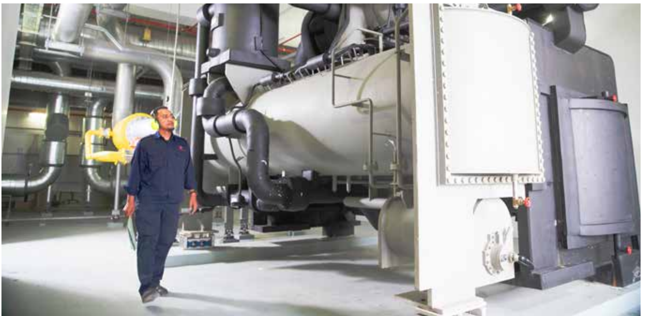
We ensure that our chiller system is always kept at optimum operating efficiency.
