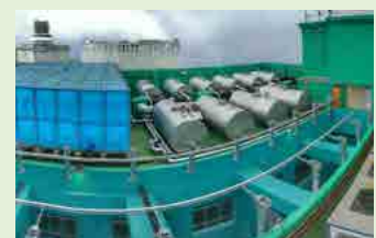
Renewable energy hot water system at FWH.
