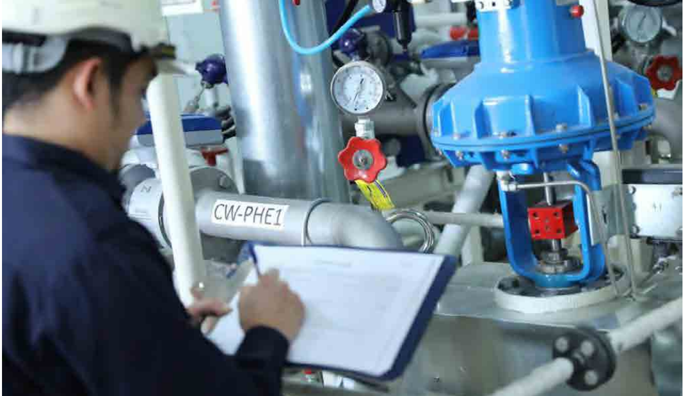
Daily inspection of plate heat exchanger ("PHE") to ensure reliability and energy efficiency of the system.
