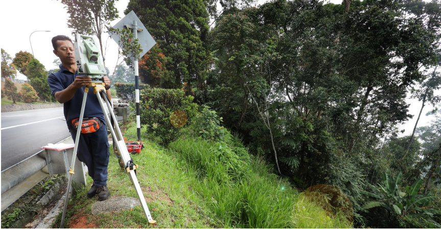
Scheduled slope monitoring by contracted surveyor to check slope movement using inclinometer
