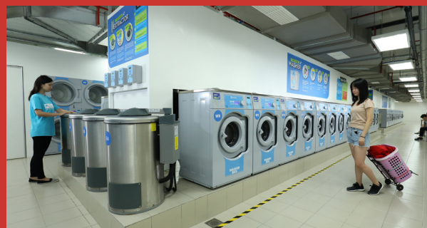
User-friendly and modern self-serving Laundry Facilities for employees
