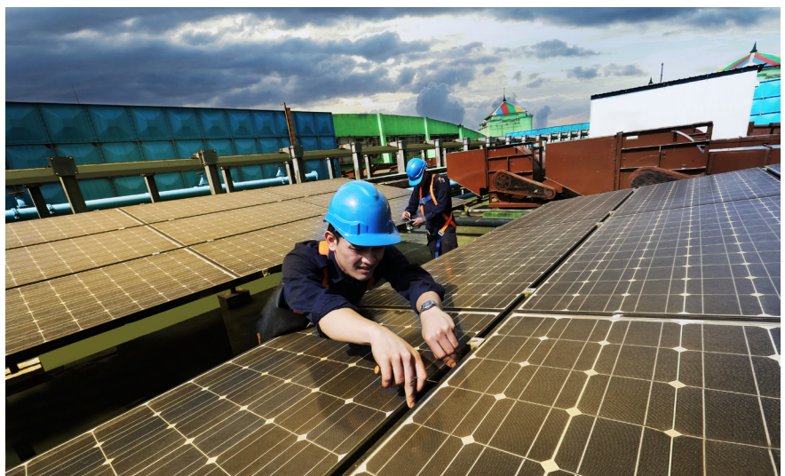
Pilot Solar Energy System Feasibility Studies
