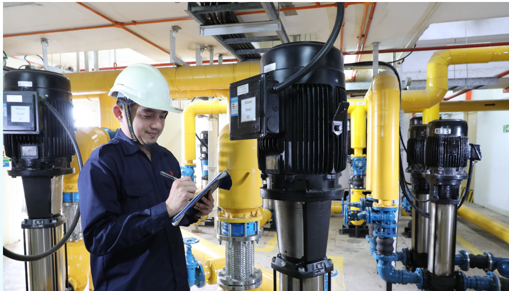
Energy Efficient Water Pump System
