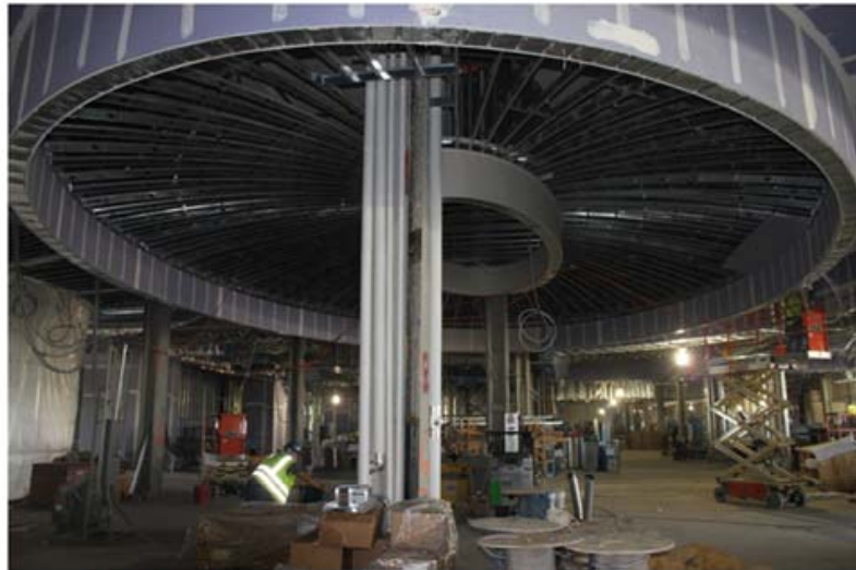
5 th Avenue Casino – Center of gaming floor ceiling feature
