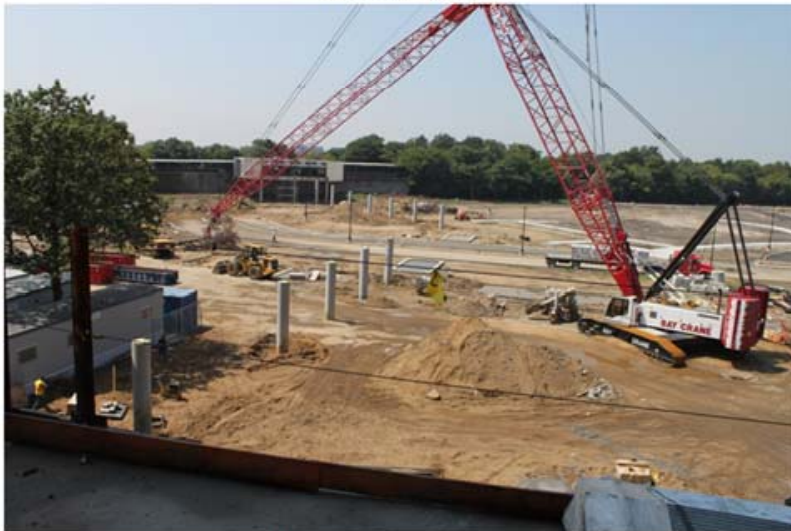
MTA Bridge Connector
