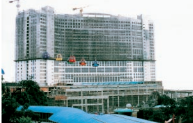
The first phase of First World Hotel under construction
